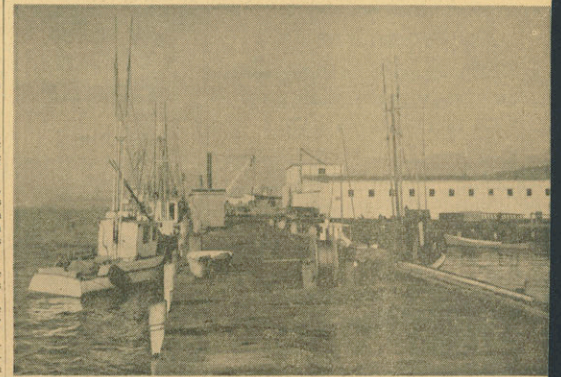
Looking toward the Norcal fish processing plant from the Paladini docks, at Fields Landing—where deep-sea vessels discharge their valuable cargoes.
